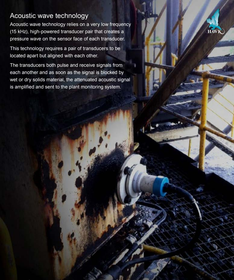
The low frequency, high power applied to the sensors also has a self-cleaning feature when the pressure wave is created. This pulsing pressure wave keeps material from adhering to the face and provides for maintenance-free operation in critical applications.
