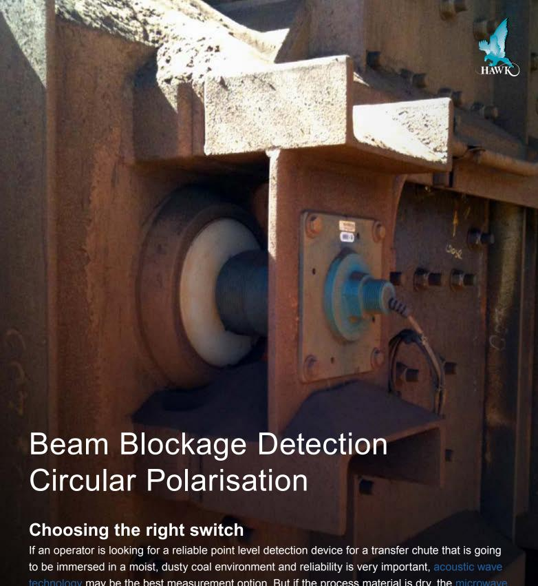
technology may be the best measurement option. But if the process material is dry, the microwave detection switch may be the best choice.
