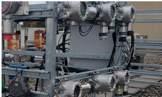
Each of these sensors, sixteen H<sub>2</sub>S sensors and fourteen CO sensors, were calibrated prior to installation and have been intermittently gas tested to verify response. No calibrations have been conducted on any of these sensors for over three years and Adaptive Environmental Compensation (AEC) has been testing the sensor every six hours and adjusting sensor response to account for changes in its sensitivity due to environmental conditions and sensor degradation.
